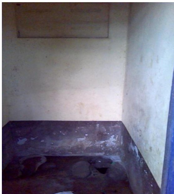
Figure 4.4 Pit Latrine at Ghana National Basic
