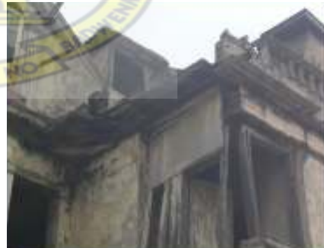
Fig.32 Broken slab of the upper terrace
