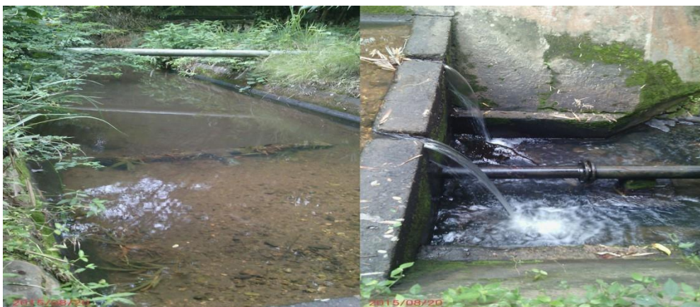
Figure B. 1 The dammed section on River Taale with its distribution pipes
