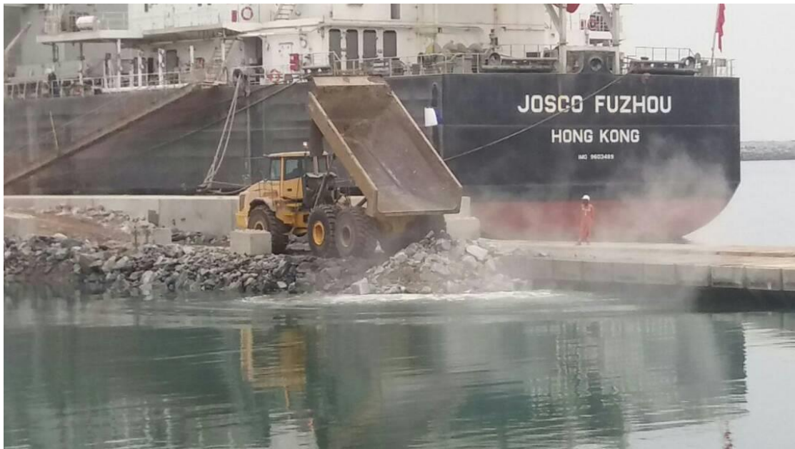
Picture showing bolders to support the side of the keywall
