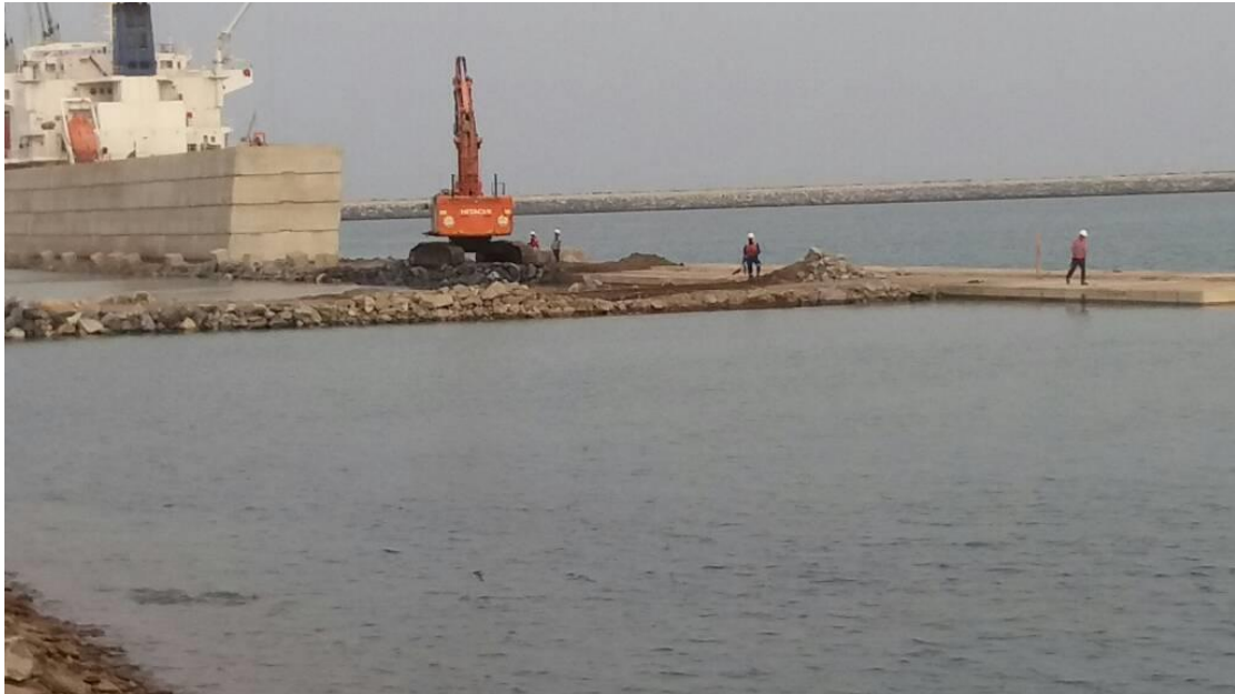
Picture showing placing of bolder and leveling with payloader
