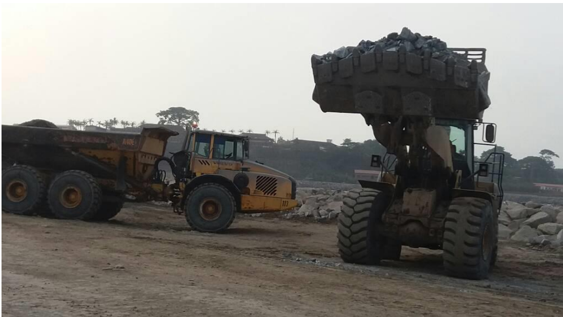
Picture showing the spreading of bolder along the key wall
