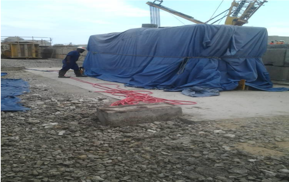
Picture showing curing process of precast blocks
