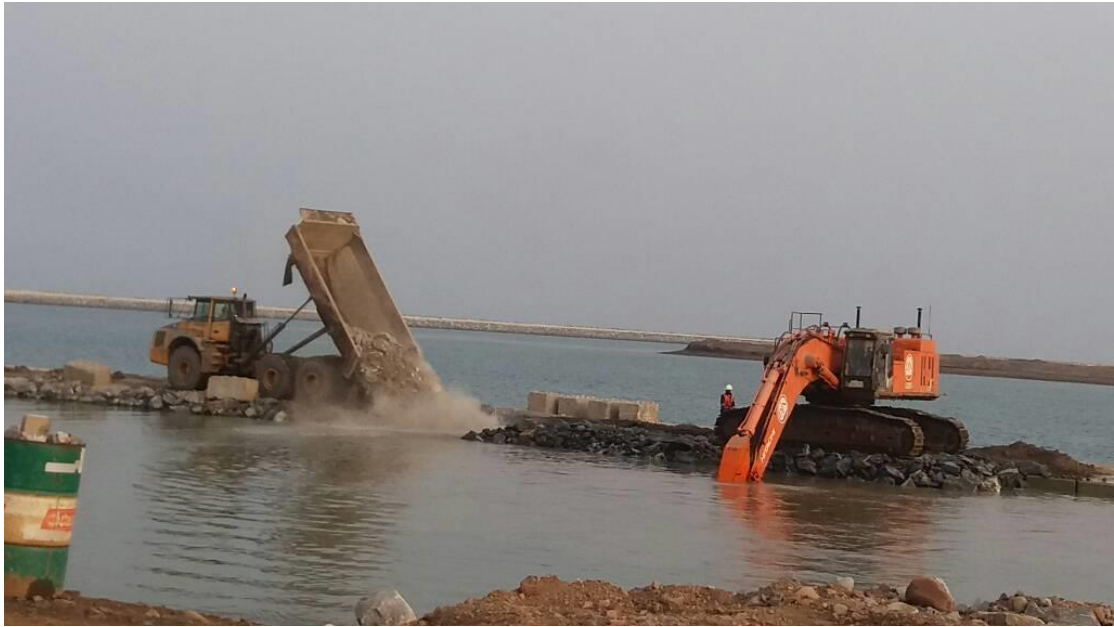
Picture showing placing and positioning bolder with excavator
