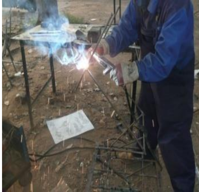
Fig. 3.90: welding the armature
