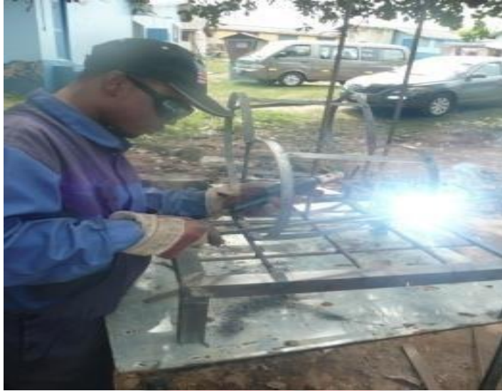
Fig. 3.53: depicts the welding of the horizontal reinforcement and the vertical iron rods for the main armature.
