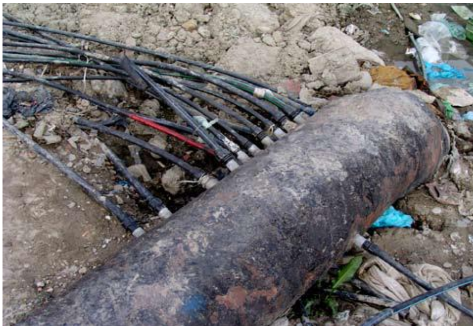
Figure 2-3: Illegal Connection
