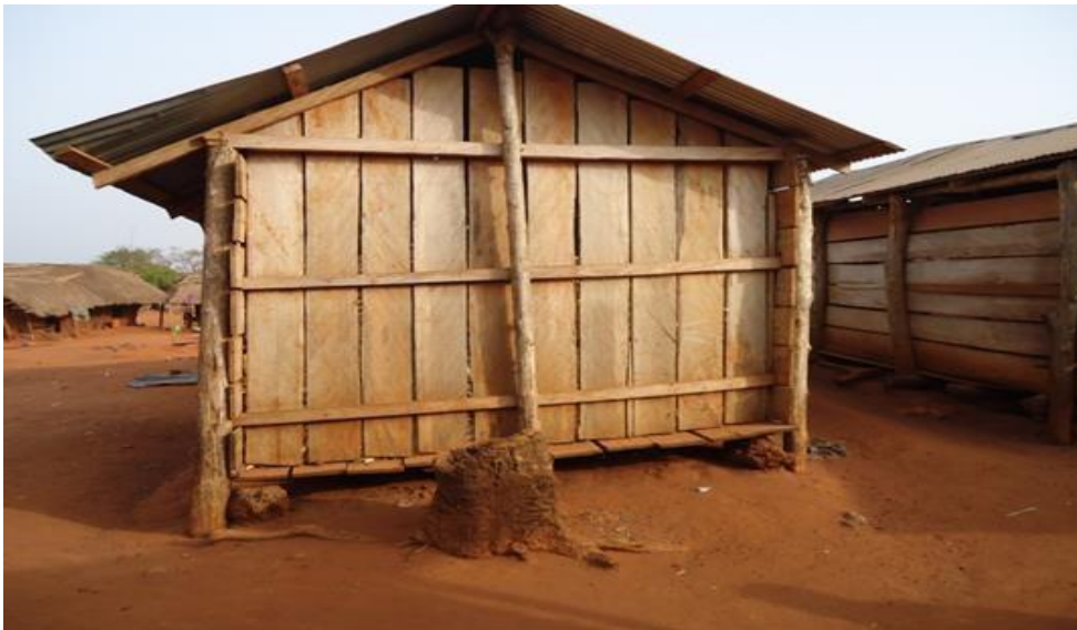
Figure. 4.5 Wider crib (WC) for maize storage
