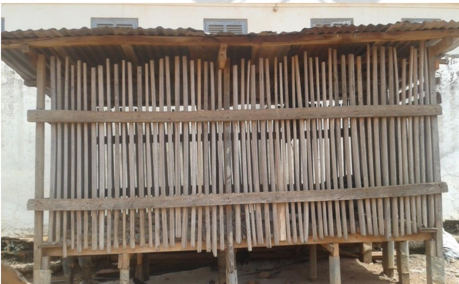
Figure 4.6. Narrow crib (NC) for maize storage
