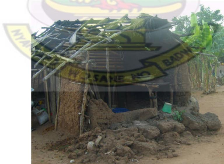
Figure 1.1 *Rammed earth house in the deteriorated state*
