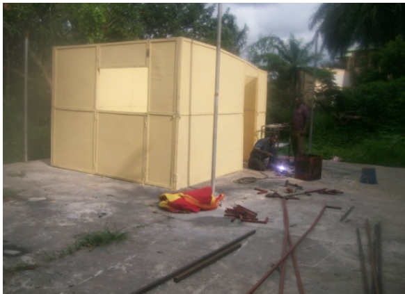
Welding the Metal Bars
