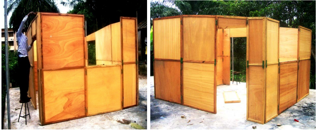
Figure 106. The Erection Process
