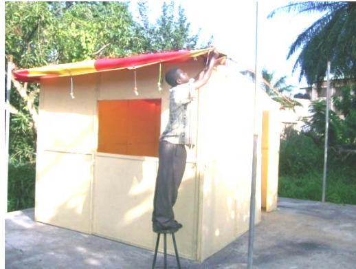
(1) Roofing with the tarpaulin
