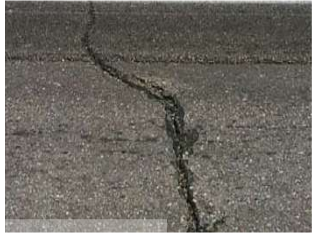
Figure 2.24A: High Severity Transverse cracks
