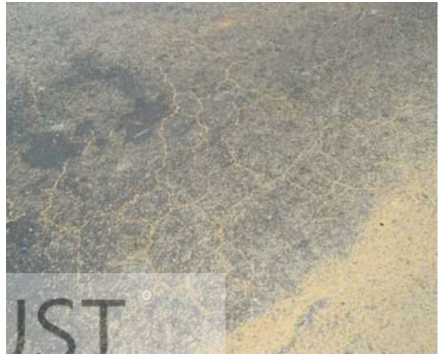
Figure 4.7: Ravelling with fatigue crack
