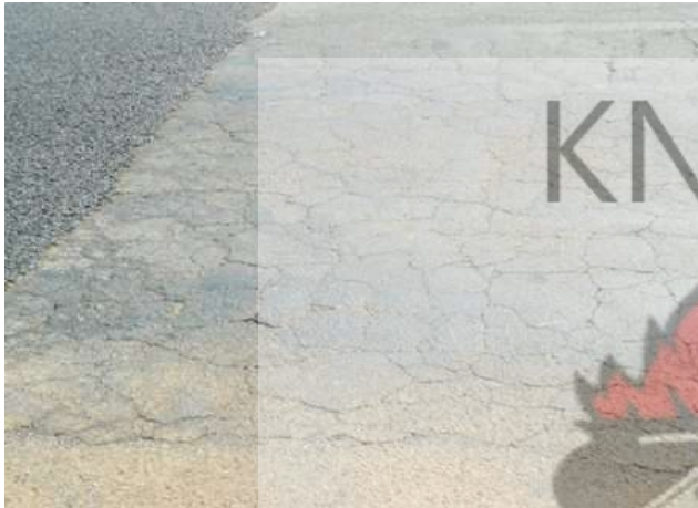
Figure 4.23: Severe Alligator cracks on a Patch
