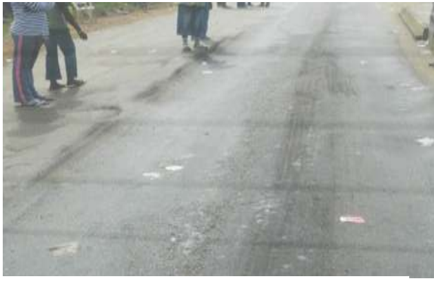
Figure 4.21: Severe Shoving and Rutting
