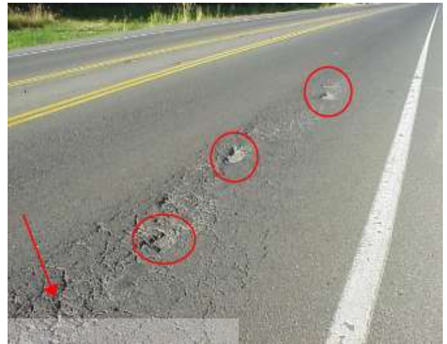
Figure 2.6A: High severity fatigue cracking
