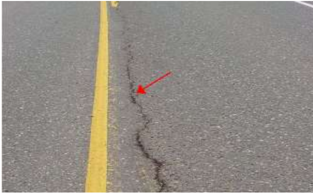
Figure 2.17A: Medium Severity Longitudinal cracking Figure 2.18A: High Severity Longitudinal cracking
