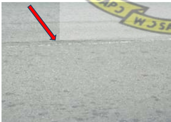
Figure 4.10: Cracking at Asphalt
