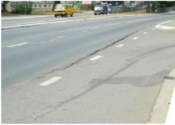
Figure 4.3: Shoving along a wheel path
