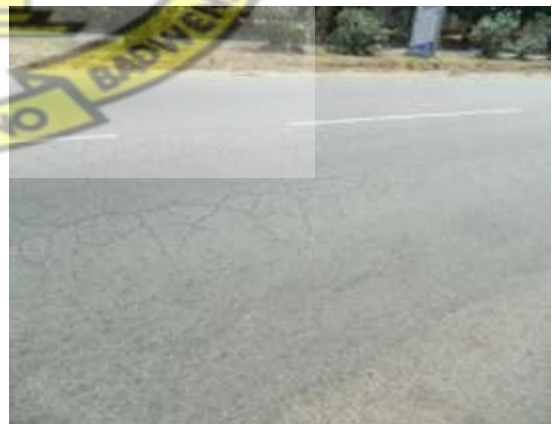
Figure.4.2: Alligator cracks
