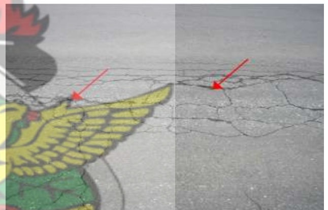
Figure 2.8A: Moderate severity Alligator cracking
