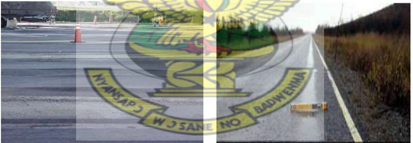
Figure 2.3A: High severity rutting on Asphalt
