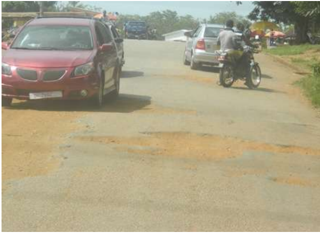
Figure.4.27: Severe Potholes at Mankranso bypass
