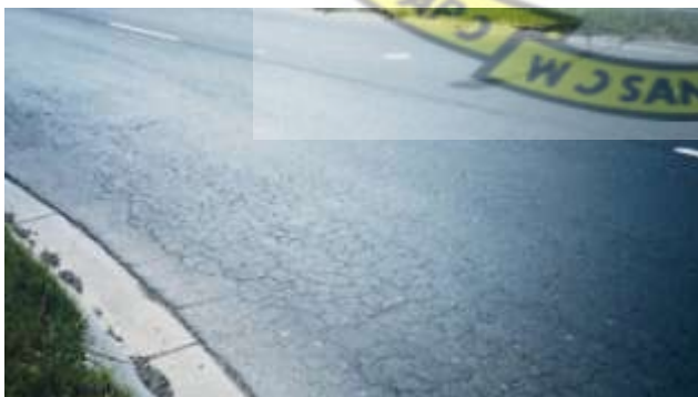
Figure 2.9A: High severity Alligator cracking
