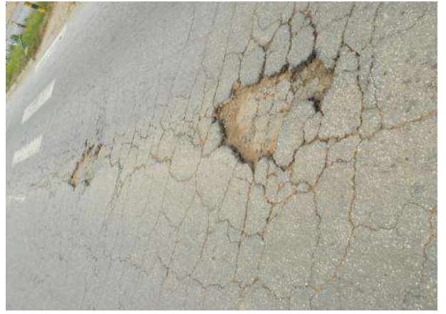
Figure.4.42: Severe Alligator cracks with Potholes
