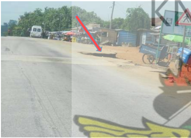
Figure 4.29: Severe Shoulder damage
