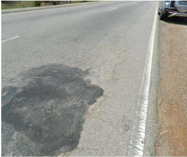
Figure 4.12: Deformation patch
