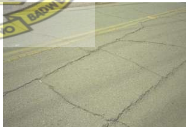
Figure 2.16A: High Severity Block cracking
