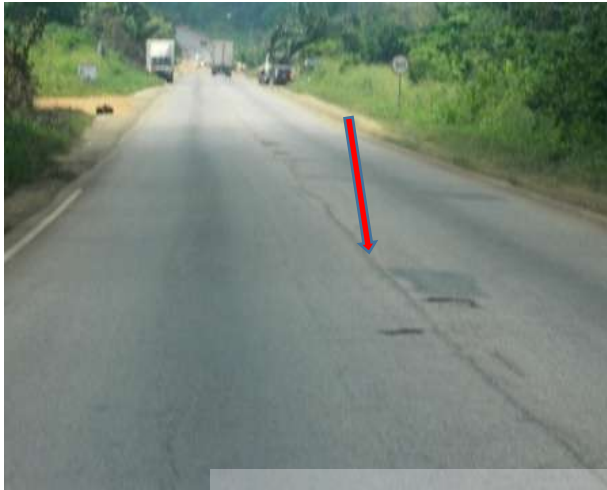
Figure 4.33: Moderate Longitudinal cracks
