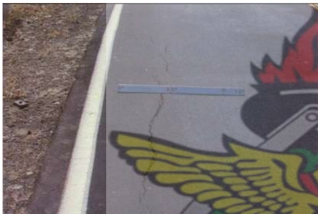
Figure 2.19A: Low Severity Longitudinal cracking Figure 2.20A: High Severity Longitudinal cracking
