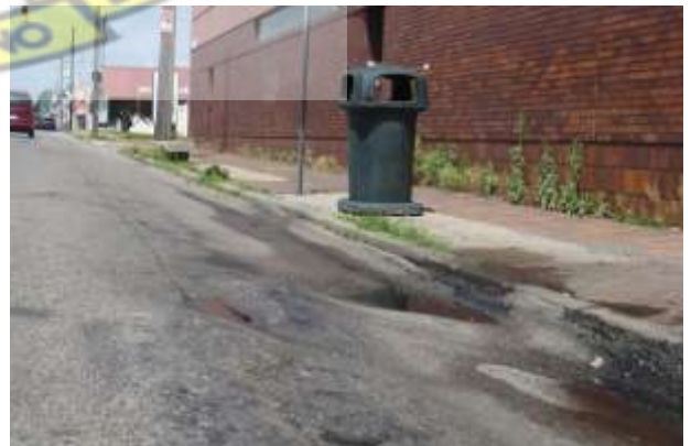
Figure 2.32A: High Severity Shoving
