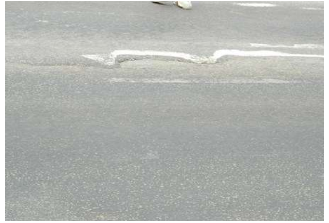
Figure 4.36: Severe Shoving (close up)
