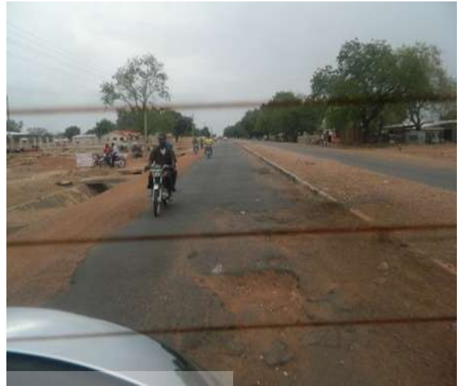
Figure 4.17: Edge cracks, shoving and potholes
