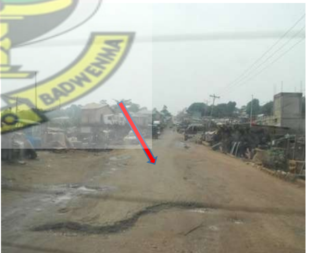
Figure 4.46: Very Severe Surface deformation
