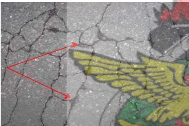
Figure 2.7A: Moderate severity Alligator cracking
