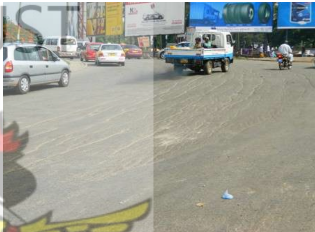
Figure 4.44: Slippage cracks with moderate Ruts
