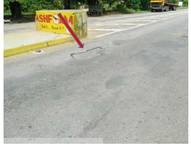
Figure 4.34: Low Severity Shoving and Pothole
