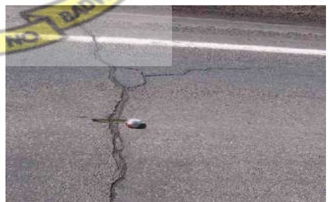
Figure 2.22A: High Severity Transverse cracking
