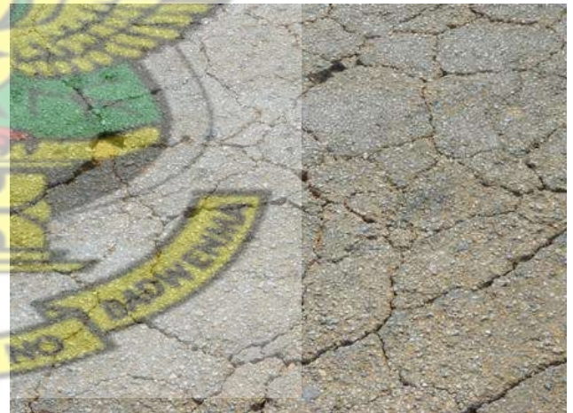
Figure 4.26: Alligator cracks (close up)
