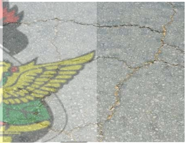
Figure 4.9: Block Cracks
