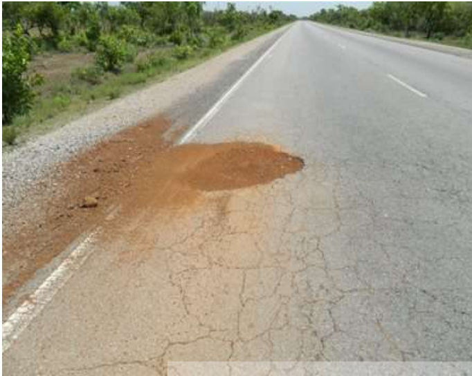
Figure 4.16: Pothole
