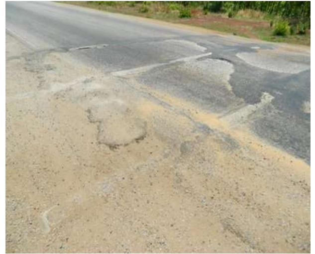
Figure 4.13: Deformation at a ramble strip
