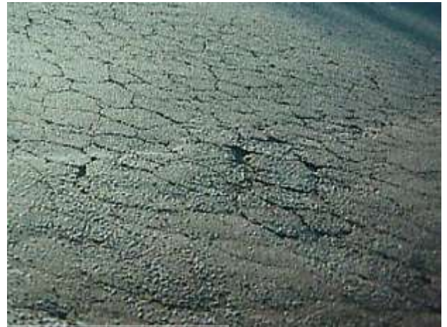
Figure 2.12A: High severity Alligator cracking
