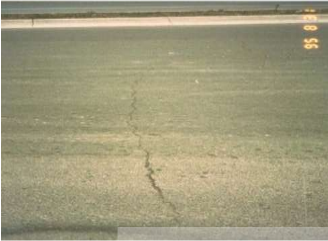
Figure 2.23A: Medium Severity Transverse cracking
