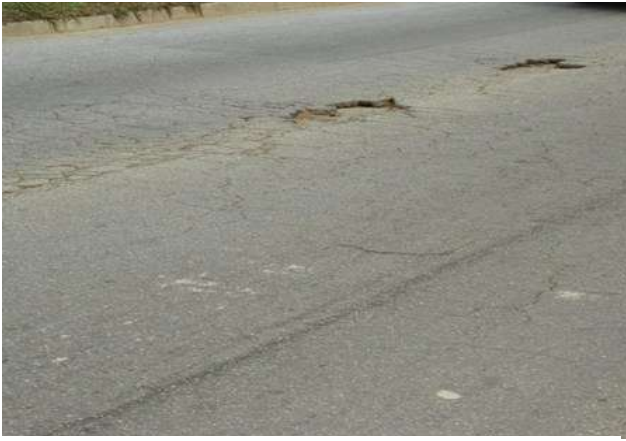
Figure 4.41: Alligator cracks with Potholes
