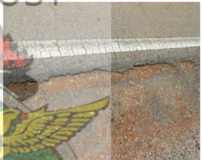
Figure 4.15: Edge Cracks
