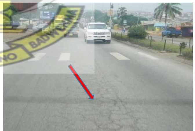
Figure 4.40: Moderate Block cracks
