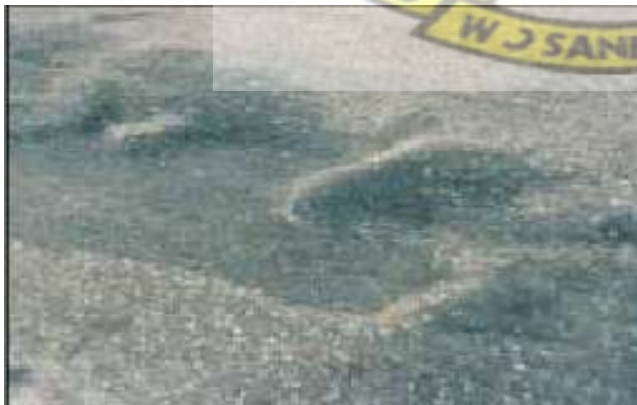
Figure 2.31A: Moderate Severity Shoving
