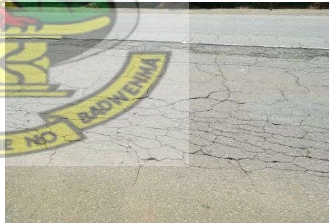
Figure 4.32: Severe Block cracks (close up)
