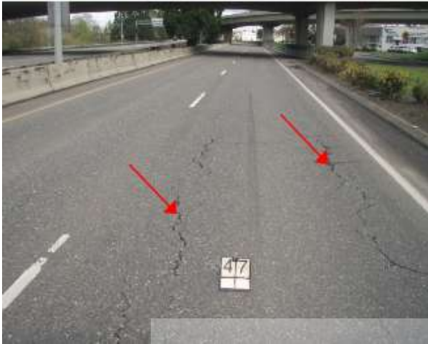
Figure 2.5A: Moderate severity fatigue cracking
