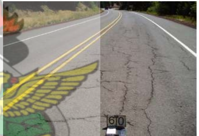
Figure 2.14A: Moderate severity Block cracking
