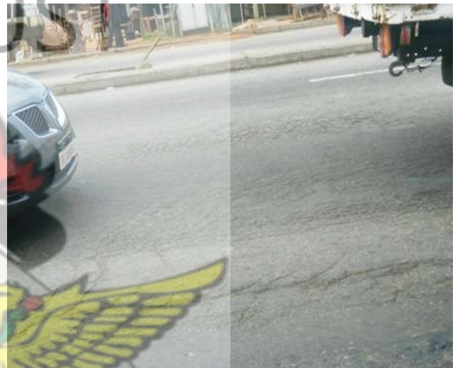
Figure 4.38: Moderate Slippage cracks
