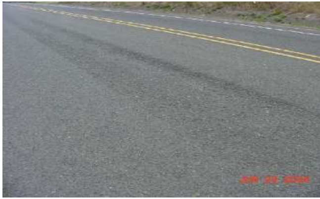
Figure 2.27A: High Severity Ravelling
