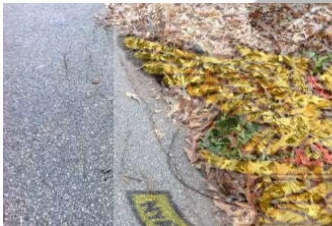
Figure 2.25A: Low Severity Edge cracks
