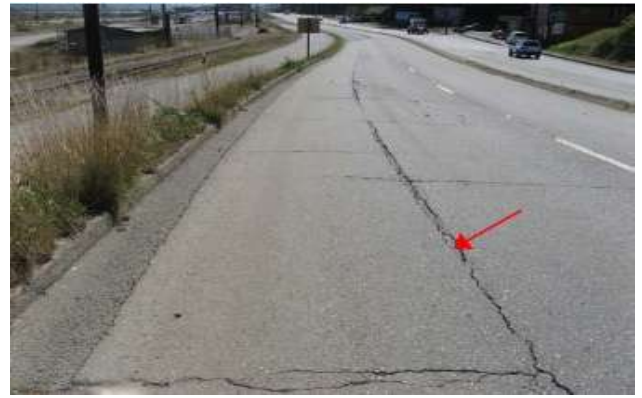
Figure 2.17A: Medium Severity Longitudinal cracking Figure 2.18A: High Severity Longitudinal cracking
