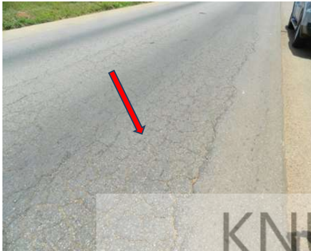
Figure 4.6: Fatigue Cracks
