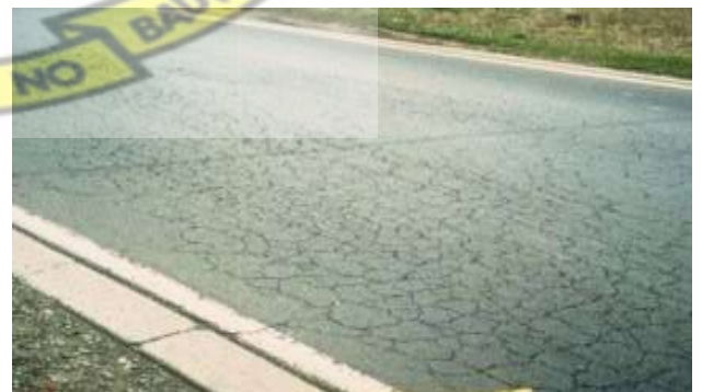
Figure 2.10A: High severity Alligator cracking
