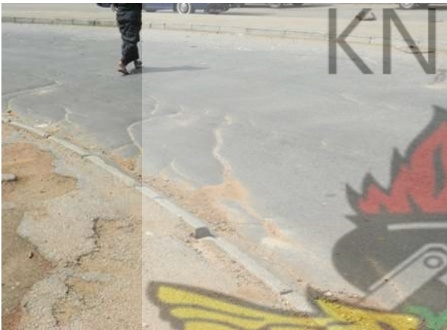
Figure 4.43: High Severity Shoving at a roundabout
