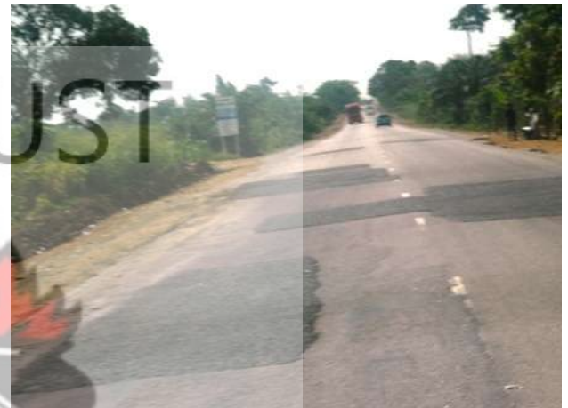
Figure 4.24: Severe Patching
