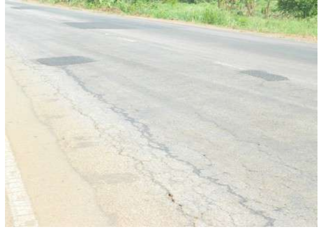
Figure 4.28: Severe fatigue cracks with patches
