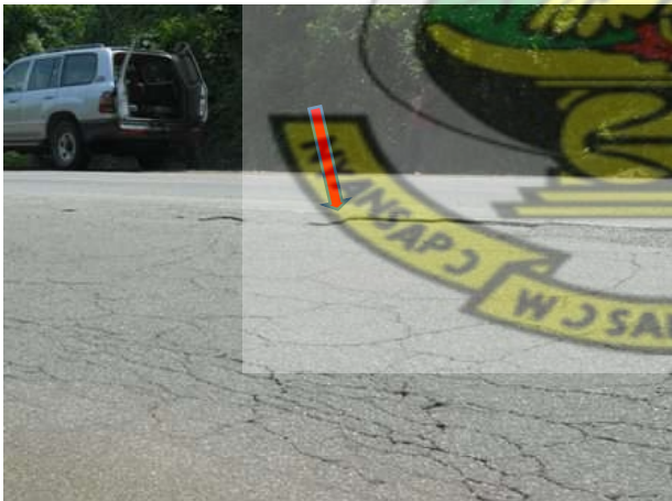
Figure 4.31: Severe Block and Seam cracks
