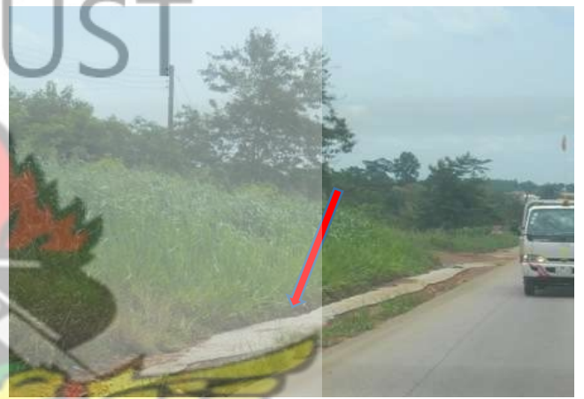
Figure 4.30: Severe Shoulder damage
