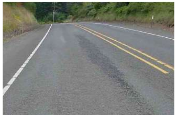
Figure 2.28A: Medium Severity Ravelling
