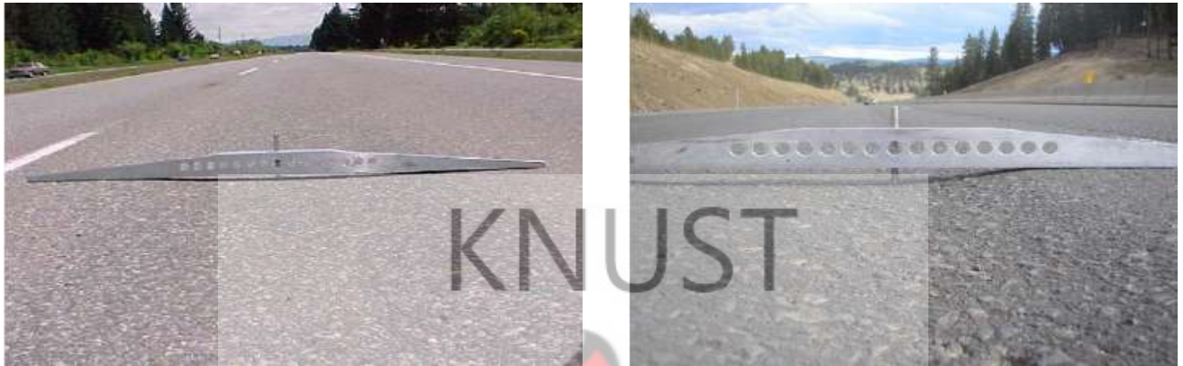
Figure 2.1A: Moderate severity rutting on Asphalt road Figure 2.2A: High severity rutting on Asphalt road
