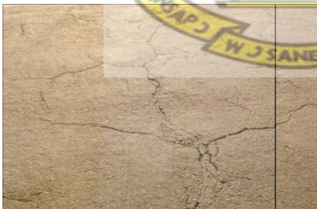
Figure 2.15A: Low Severity Block cracking
