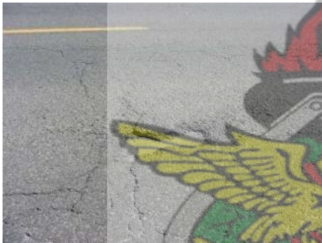
Figure 2.29A: Medium Severity Pothole
