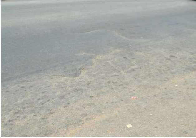
Figure 4.35: Low Severity shoving
