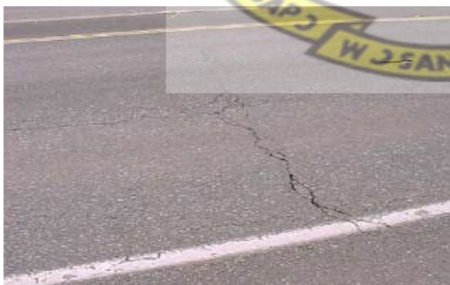
Figure 2.21A: Medium Severity Transverse cracking
