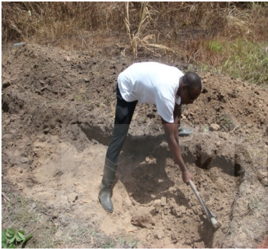
Plate 2: Digging of SSF CW
