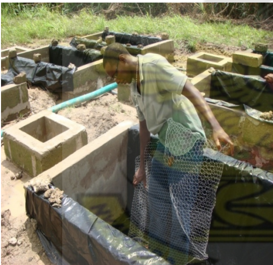
Plate 4: Installation of screens
