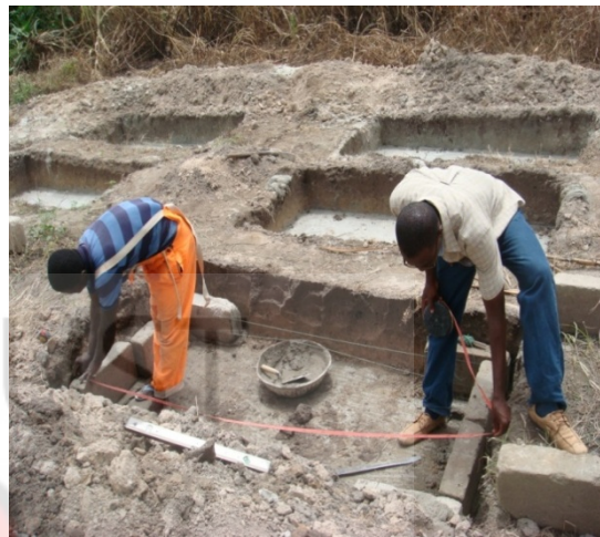
Plate 3: Construction of SFF CW
