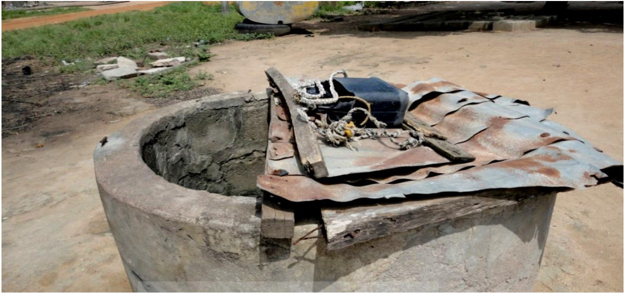
Plate 3. Photograph of Hand Dug Well 3 showing a plastic gallon container and attached rope used for fetching water from the well.
