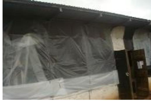
Figure 4.4 Cement block and wire mesh pen with plastic curtains for brooding
