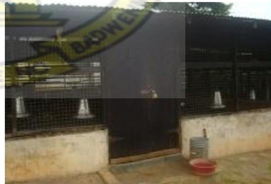
Figure 4.2 Pen with 2-4 feet foundation block and wire mesh sides
