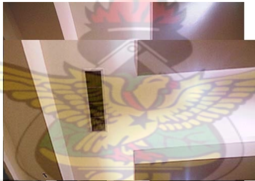
Fig.4.15. Air-condition supply outlet for the mall and shop in ASM
