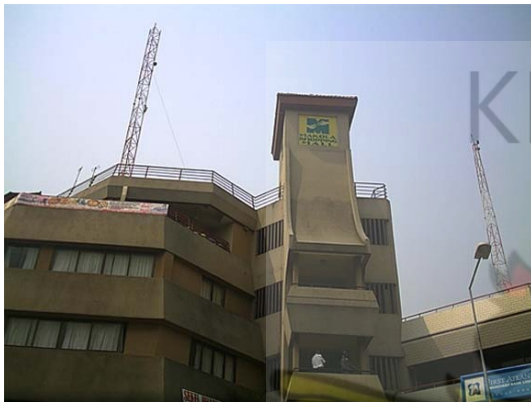
Fig.4.8. Washed terrazzo used on the facades of the office block in MSM
