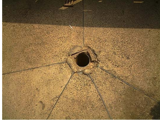
Fig.4.10. Drain gulley integrated in veranda floors of MSM
