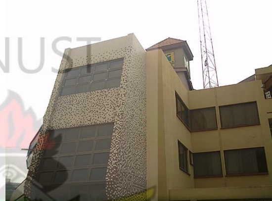
Fig.4.9. Mosaic tiles (brownish and creamish) used on the stairwell in MSM
