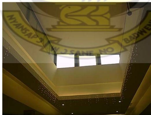
Fig.4.14. Clerestory employed to harness day lighting in ASM
