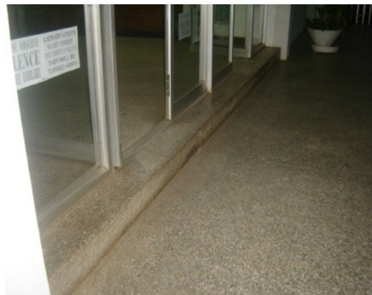
Fig.69-Raised floor level of main entrance
