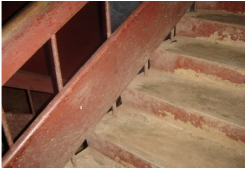
Fig.31-Un-highlighted nosings at the administration block
