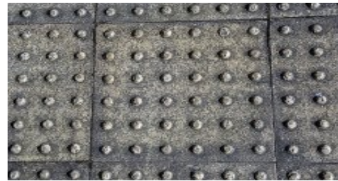
Fig.4 Embossed plate as tactile marking
