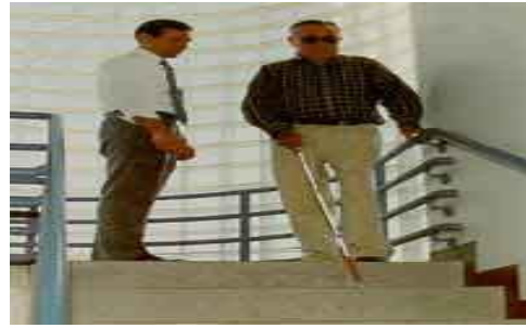
Fig.2-Handrails on both sides for support
