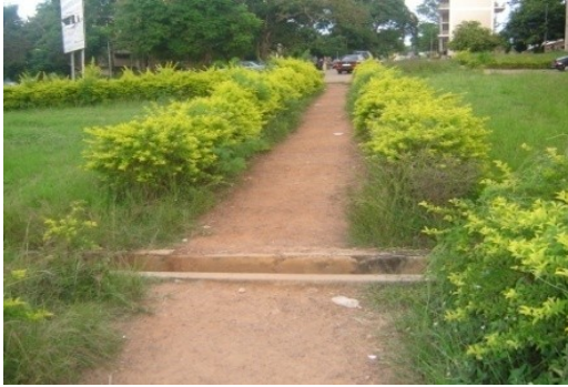
Fig.57-Gutter cutting through walkway to College of Pharmacy
