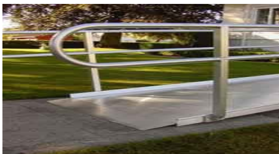
Fig.7-Handrails on the sides of an access ramp
