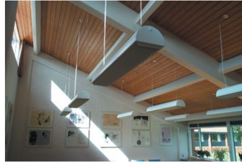
Fig.21-Ceiling design for acoustics in a classroom
