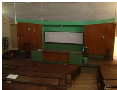
Fig.62-Wood paneling on wall to enhance acoustics
