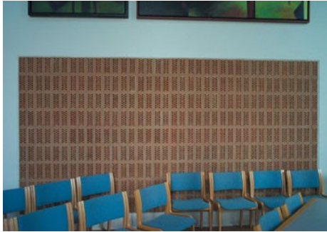
Fig.20-Brick facing at back wall for good acoustics in a classroom
