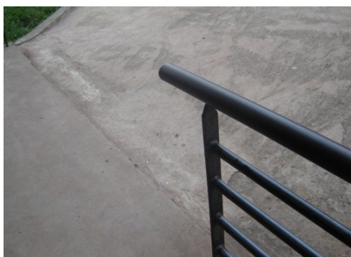
Fig.44-End of railing can be hazardous
