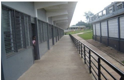
Fig.42-Metal railings on corridors of classroom block
