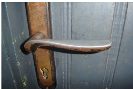
Fig.36-Simple lever handle on door
