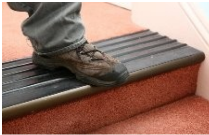
Fig.3-Tactile marking on a stair tread
