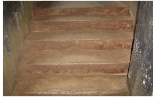
Fig.32-Un-highlighted nosings at stair of boys dormitory block
