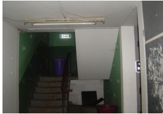
Fig.68-Stair without highlighted nosings
