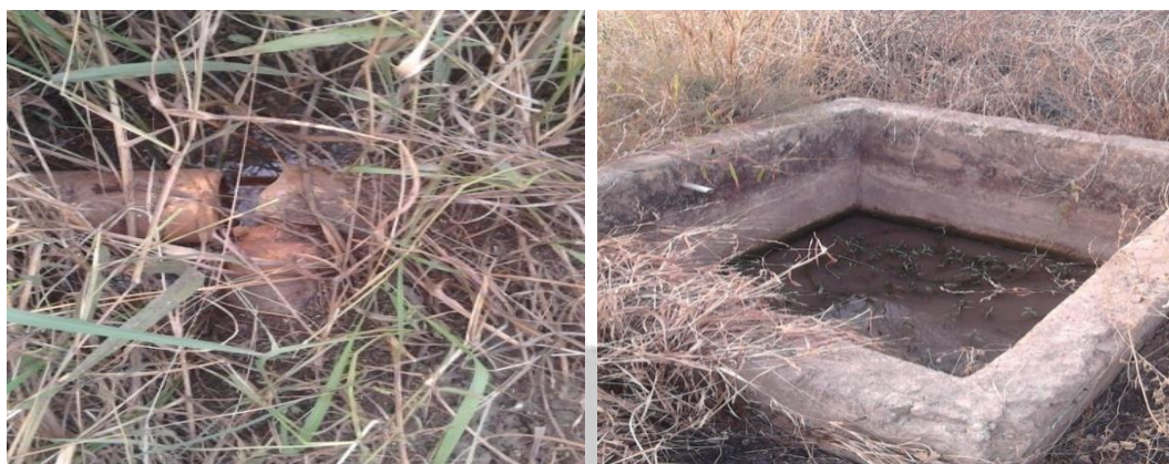
Figure 4.5: State of pipes and chambers at Kokoligu
