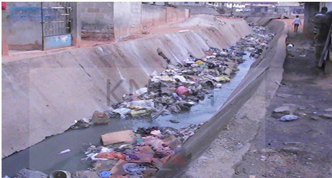
PLATE 1 Gutter choked with solid and liquid waste (Suntreso)
