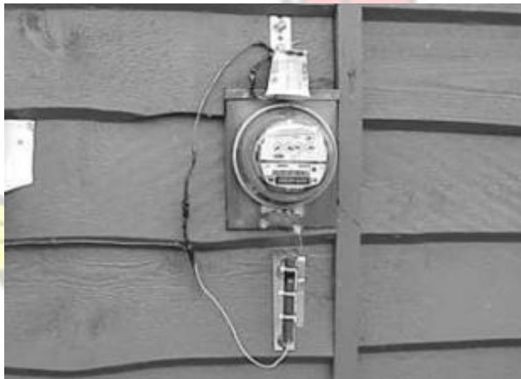
**Figure 2.13 Bypassing a meter [2.72]**
