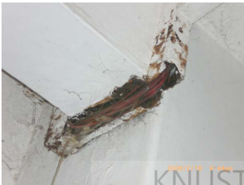
Fig 18: An exposed electrical wire in the gynaecology ward (Source: Author, February 2008)
