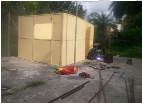
Welding the Metal Bars for the Beams/Rafts.
