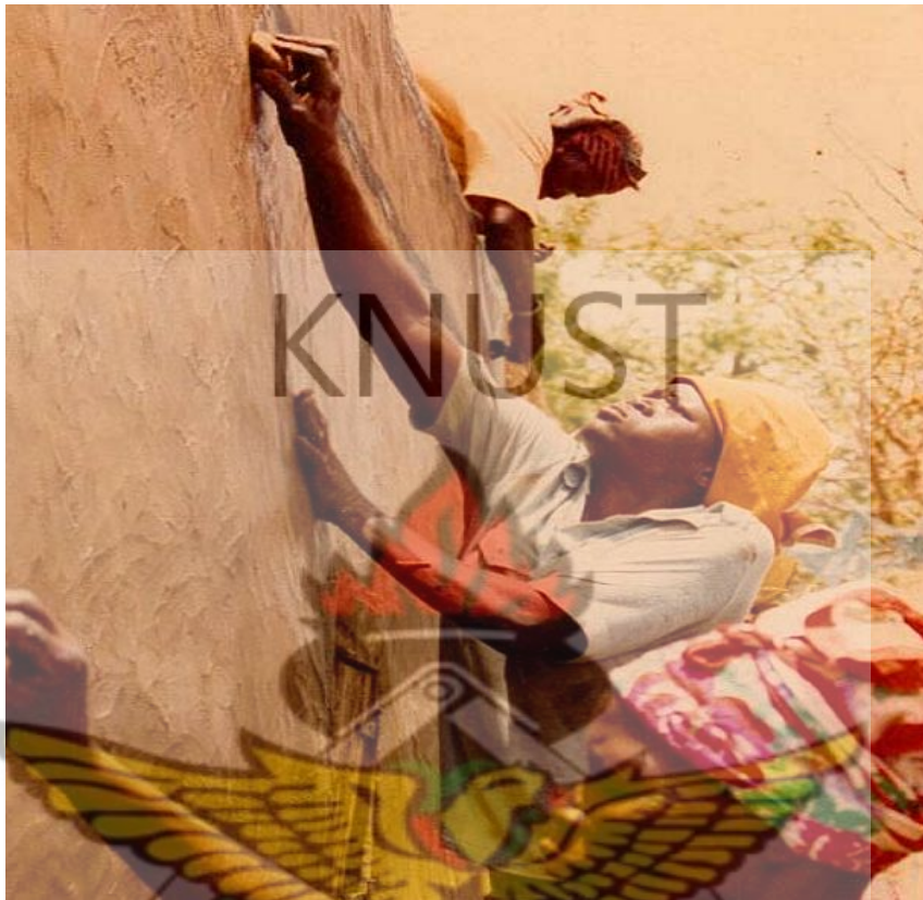
Figure 72. Women preparing surface with cold-tar plaster mixture and smoothing stones
