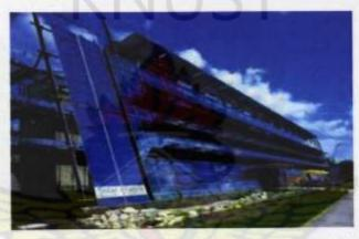
Figure 2.18: Solar fabric, Freiburg facade with transparent modules and shadowing modules
