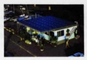
Figure 2.19: Photovoltaic system on the roof - "Les Corsaires" 7.7 kW in Switzerland
