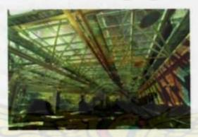
Figure 2.20: Roof integrated photovoltaic system with transparent solar modules in Switzerland
