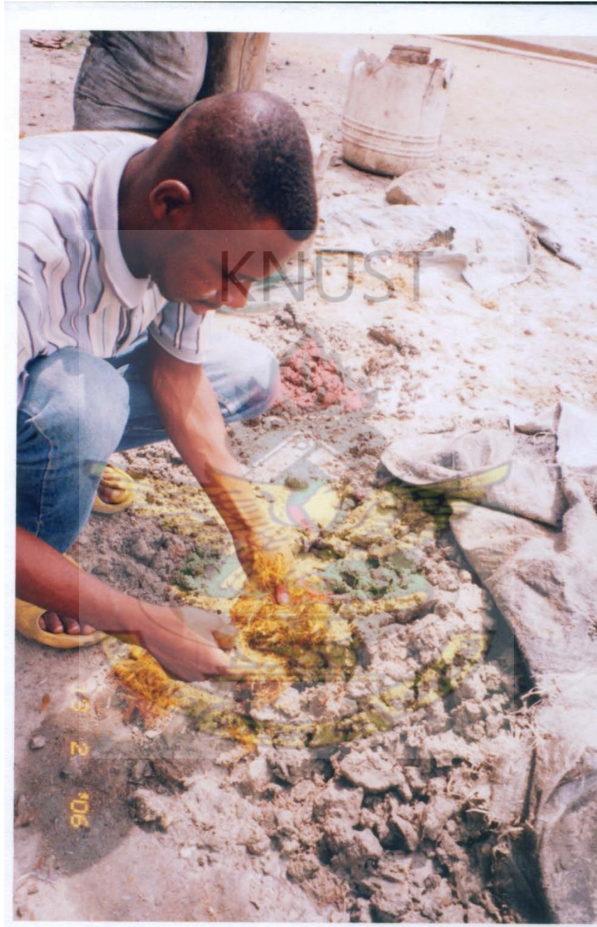
Plate 3.22 Mixing palm fruit fibre with clay to get the coarse layer (Source: Picture by researcher)
