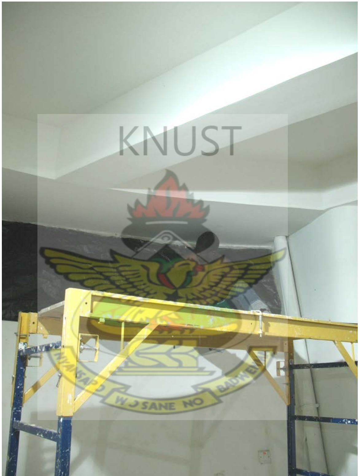
Figure 26. Blinding of light vents in preparation for Gift Shop (2008). Michael Manu-Kobia.
