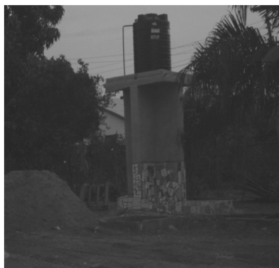
Fig.11: Borehole with stand pipe at Barekuma. Fig. 12: Borehole connected to a plastic tank. Pictures by the researcher.
