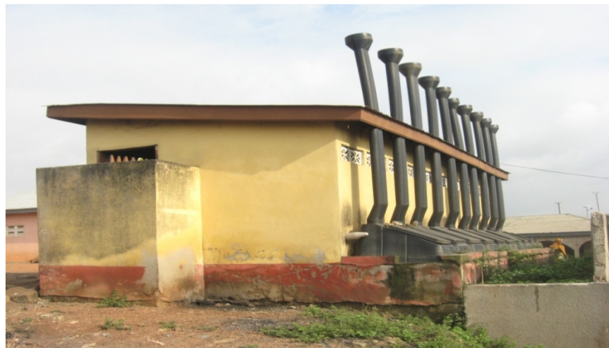
Fig. 9: Kumasi Ventilated Improved Pit (KVIP) at Akropong – picture by the researcher
