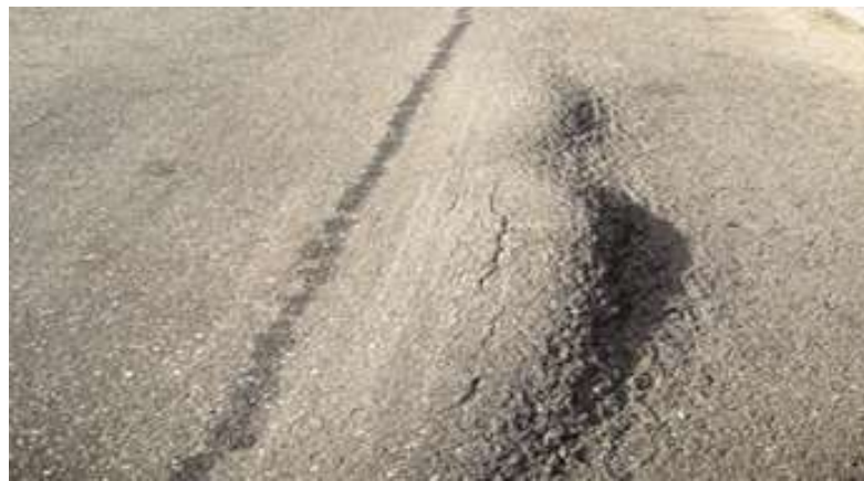
Plate 2.1. Surfacing exhibiting shoving distress
