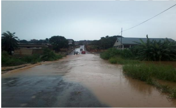
Plate 2.1. Culvert with insufficient capacity
