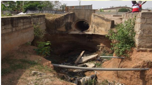
Plate 2.2. Failed culvert
