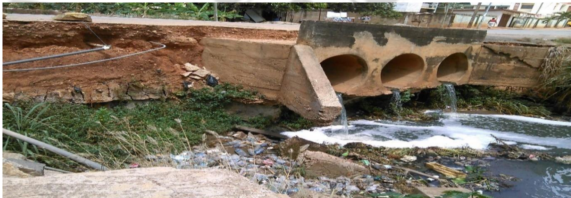
Plate 4.3: Erosion of culvert outlet
