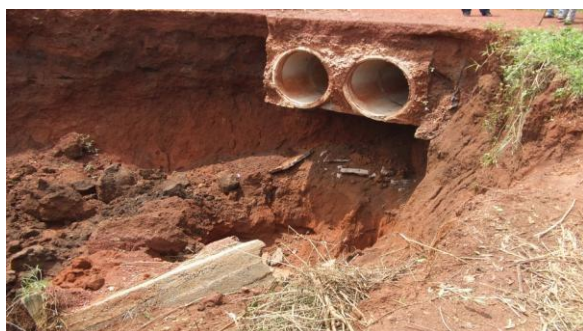
Plate 2.3. Culvert with piping failure
