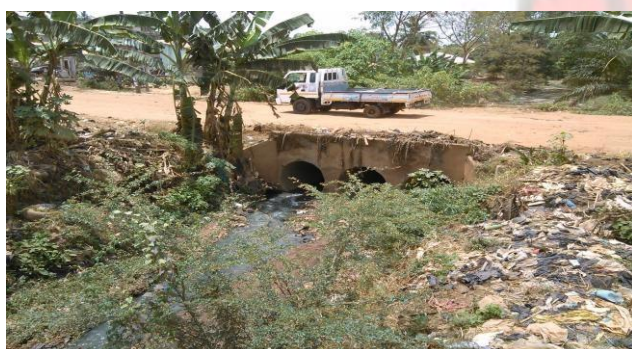
Plate 2.4 Unmaintained culvert
