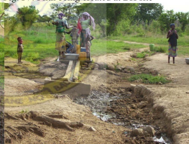
Fig. VI: Broken trough and erosion at BH site
