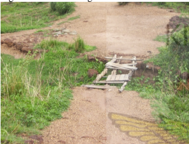
Fig. XX: Failure due to overtopping
