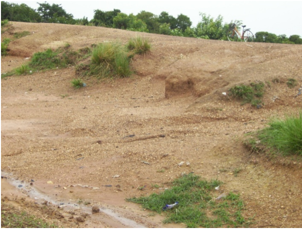
Fig. XVIII: Eroded dugout embankment
