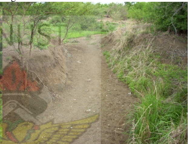
Fig. XXI: Failure due to poor compaction
