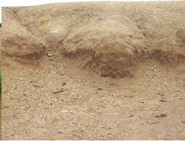
Fig. XIX: Embankment slides
