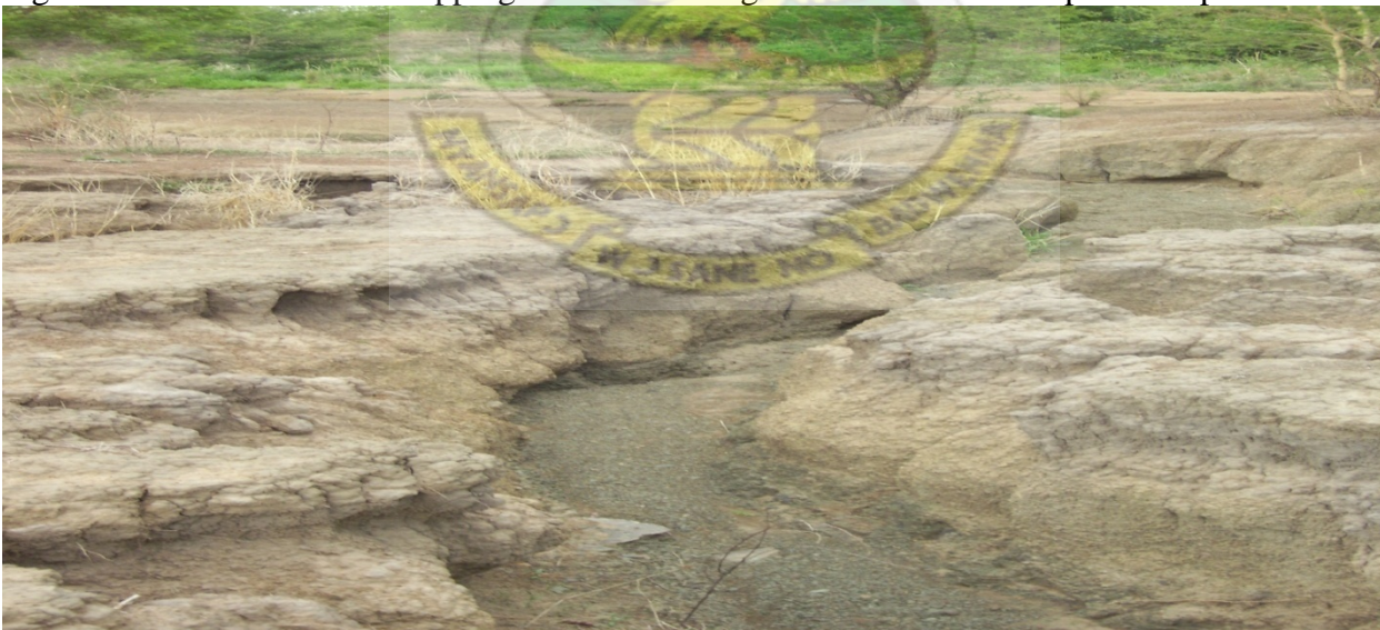
Fig. XXII: Eroded dugout embankment
