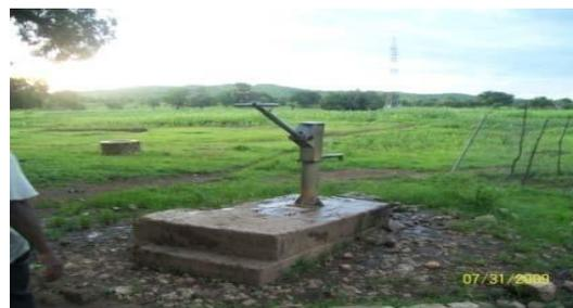
Plate 2 -2: Borehole with hand pump
