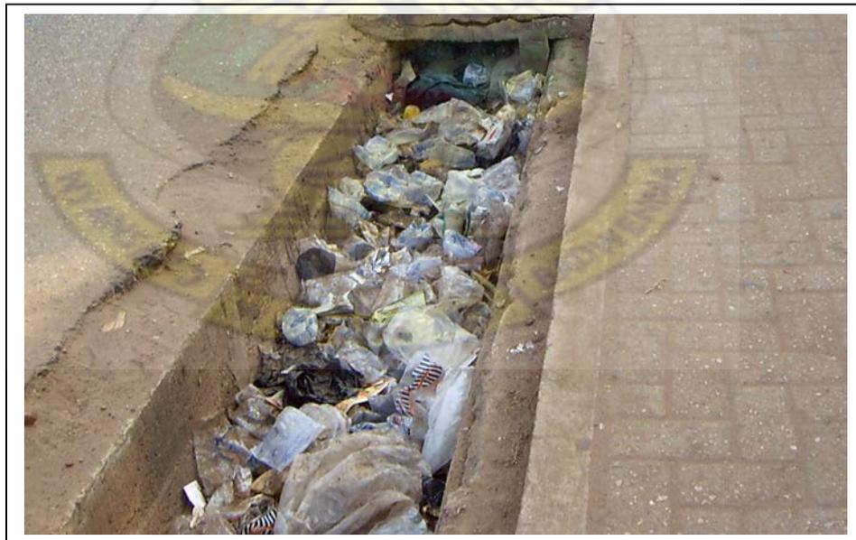
Fig. 5.12 Plastic waste choking drains and gutters near Department of National Lotteries in Central Accra
