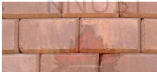
Figure 2.14 Laid interlocking stabilized soil block (Source: UN-HABITAT/Adrian Perez, 2008)
