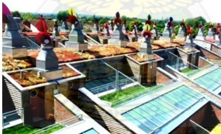
Figure 2.22 PV panels on the roof and the roof ventilators (Source BedZED Eco-Village 2008)
