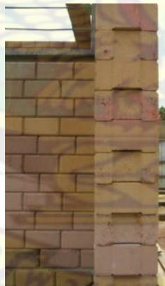
Figure 4.10 Stabilized compressed earth blocks
