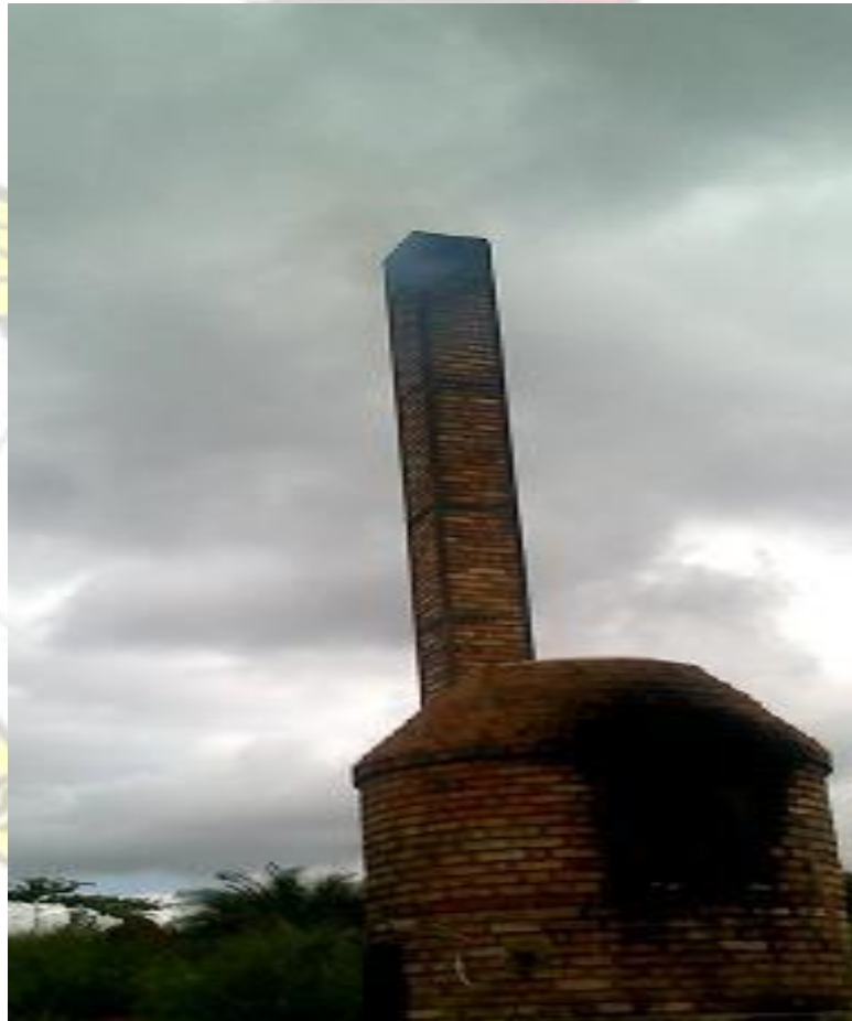
Figure 2.2 An Nsiah CT5 circular domestic incinerator at Ada Foah in the Greater Accra Region, showing black smoke emission
