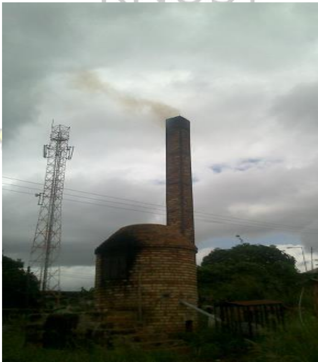
Figure 2.4 An Nsiah CT5 incinerator at Old Tafo Government Hospital in Kumasi showing black smoke emissions.
