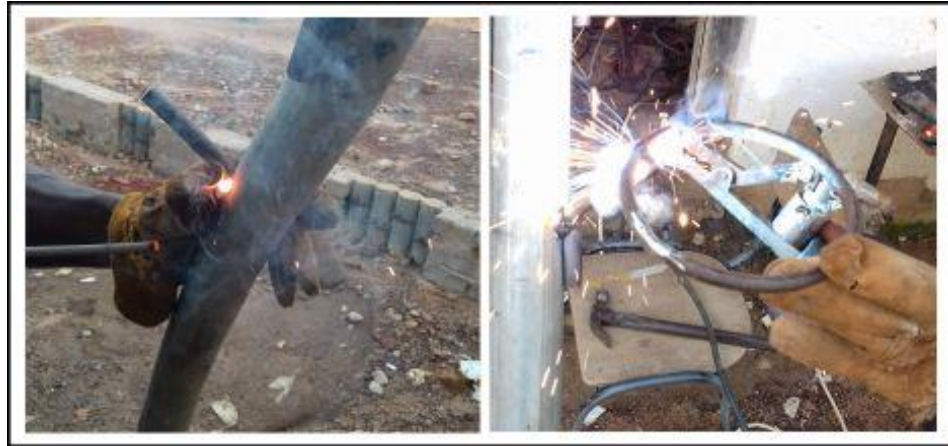
Plate 3.91: Welding the extensions to the pipe
