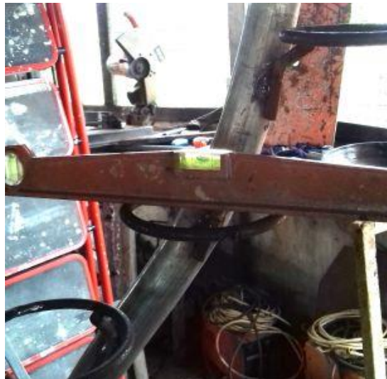
Plate 3.92: Checking for alignment
