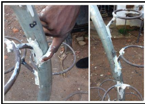
Plate 3.94: Covering the cavities with filler
