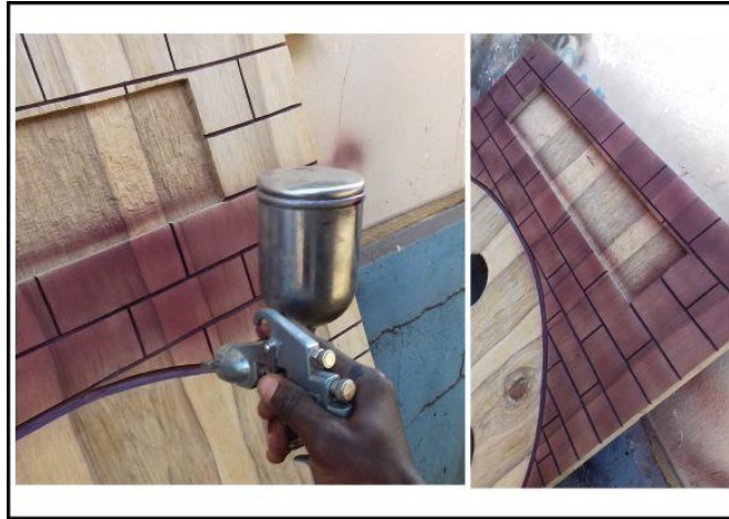
Plate 3.71: Shading the upper section.
