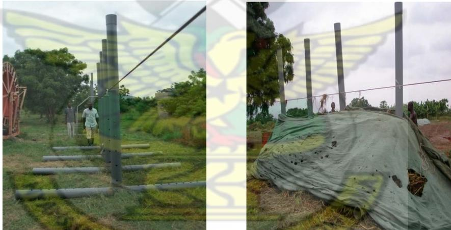
(a) Perforated uPVC pipes for HV system (b) HV set-up pile covered
