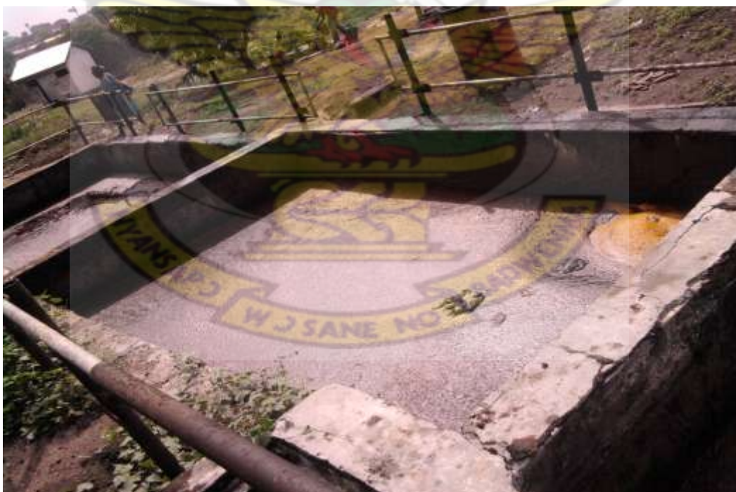
Plate B.6: Palm Oil Mill Effluent digestion tanks at a local oil mill
