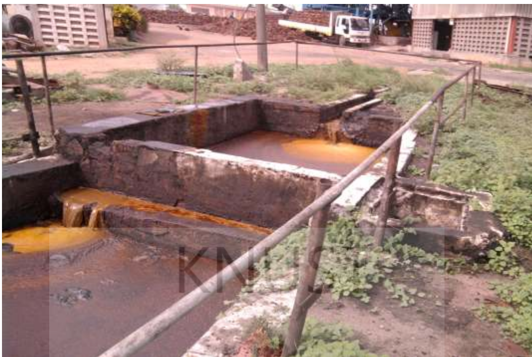
Plate B.5: Palm Oil Mill Effluent digestion tank at the local oil mill in a bad shape
