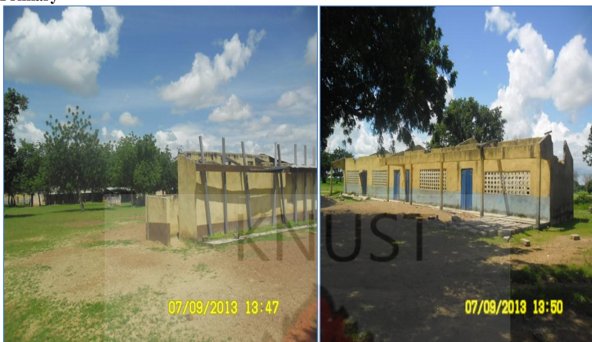
Plate 4.7: A 3-classroom block and a toilet building destroyed by windstorms in Sirigu Primary
