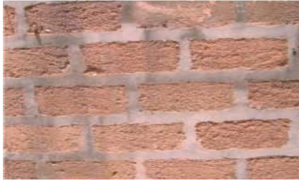
Figure 2.6 stabilized adobe wall, maintenance workshop K.N.U.S.T.
