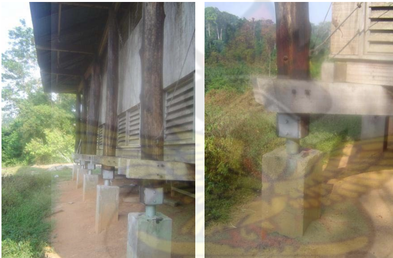
Fig. 4.11 Teak columns supported with concrete piers with floor beams bolted to teak columns.
