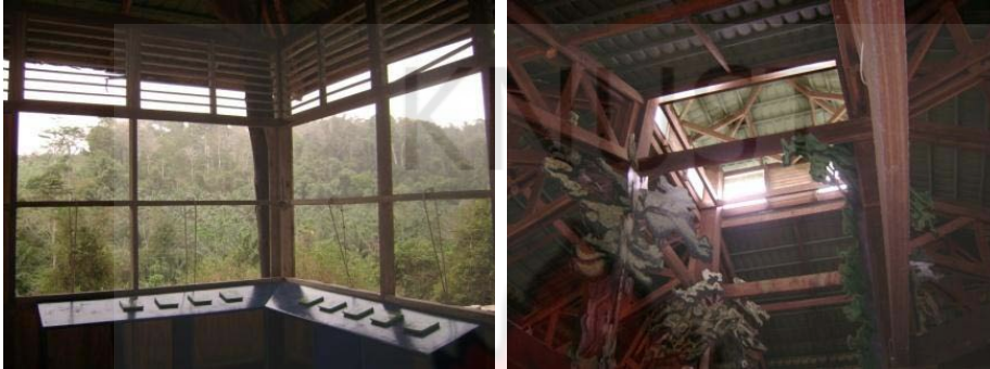
Fig. 4.9 Wide openings with sky lighting provides very high levels of day lighting in the exhibition area
