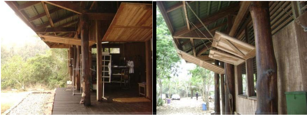
Fig. 4.12 Top Hung Doors And Windows Operated By A Pulley System
