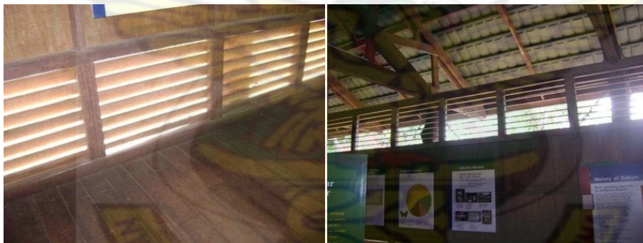
Fig. 4.8 Fixed jalousie windows at the top and bottom of the walls provide cross ventilation while leaving the middle portion for exhibits.
