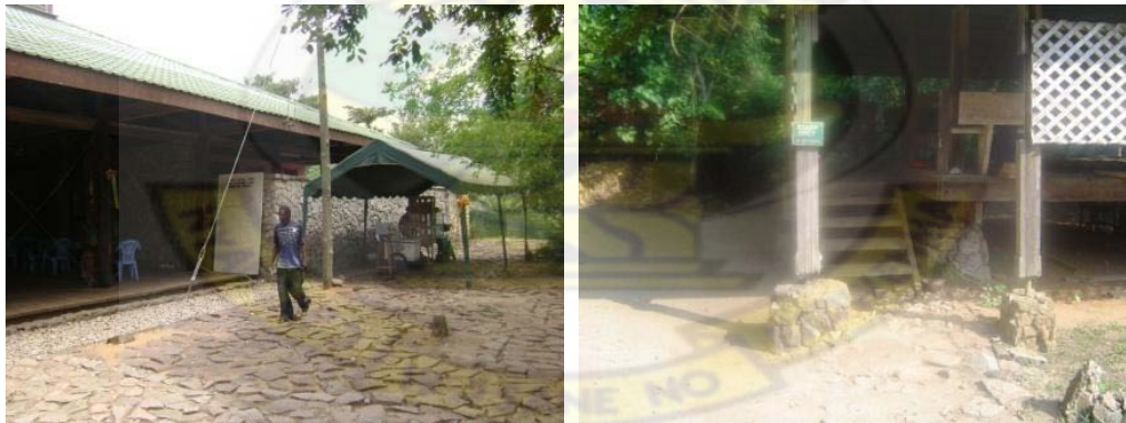
Fig. 4.10 Stone used for ground pavement, wall and pier to support column
