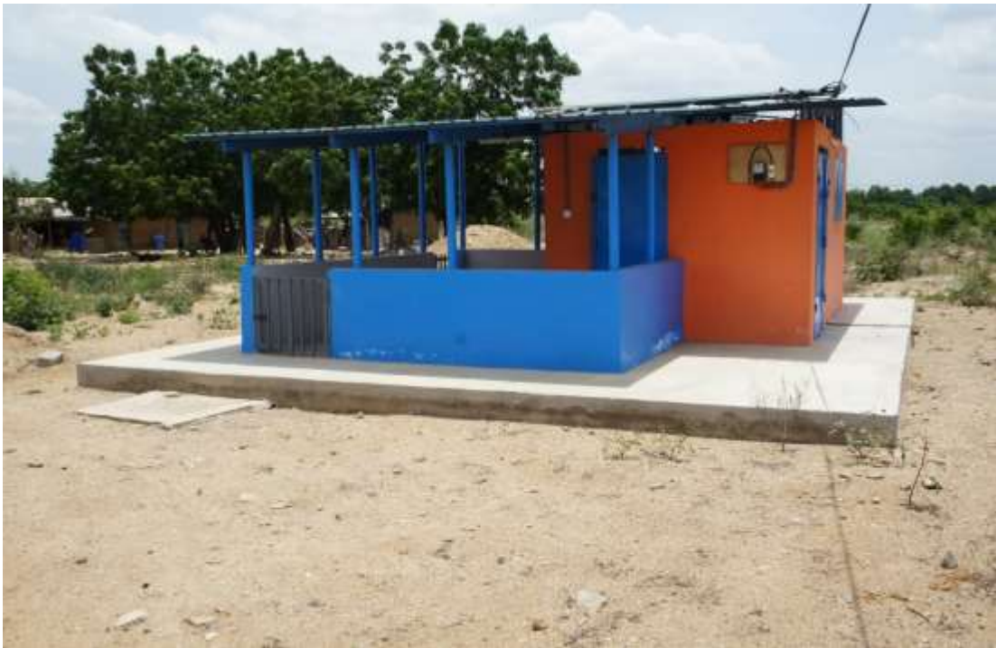
Figure 4.9: Picture of Kasunya Water Project.
