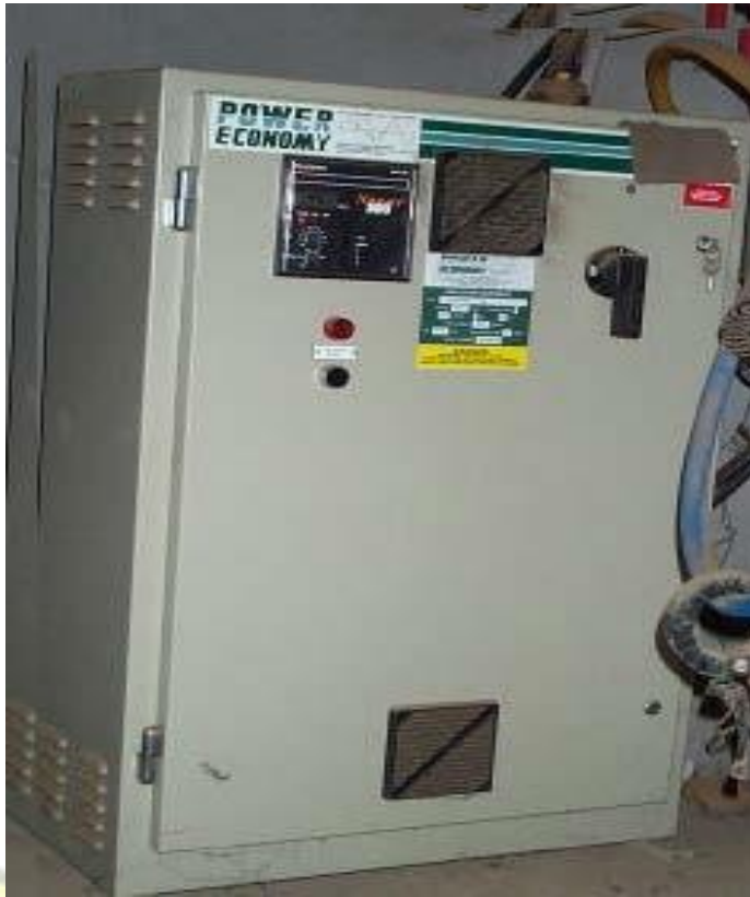
Figure 2: Power factor improvement by installation of capacitor bank (Source Energy Foundation, 2000)
