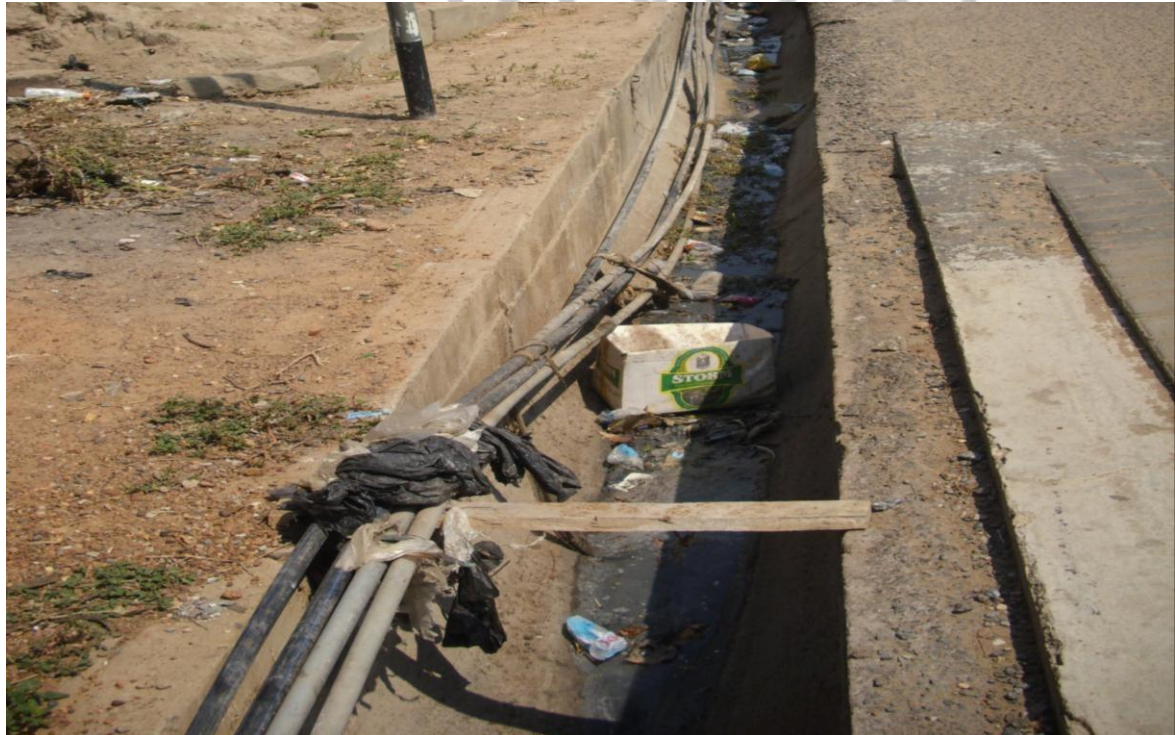
Plate 5.1: Distribution Lines in Gutters at Akweteman
