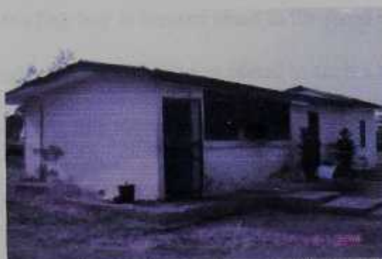
Figure 35. Kitchen and Store Area (Source: Bomarts Farms Limited – Nsawam)
