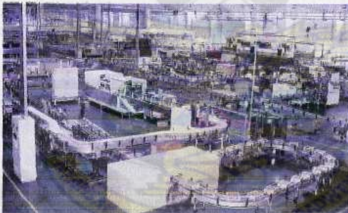
Figure 1: Food Processing Lines (Source: Korea Association of Machinery Industry)
