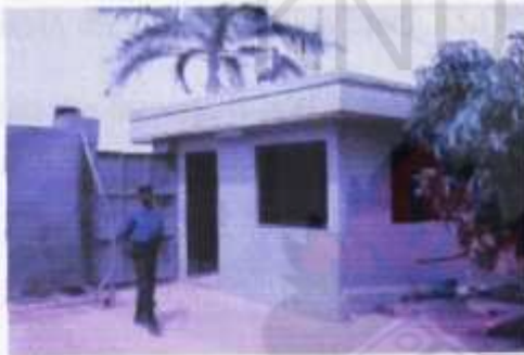
Figure 46. Entrance Gate / Security Post (Source Papso Ghana. Ltd – Off Spintex Road Accra)
