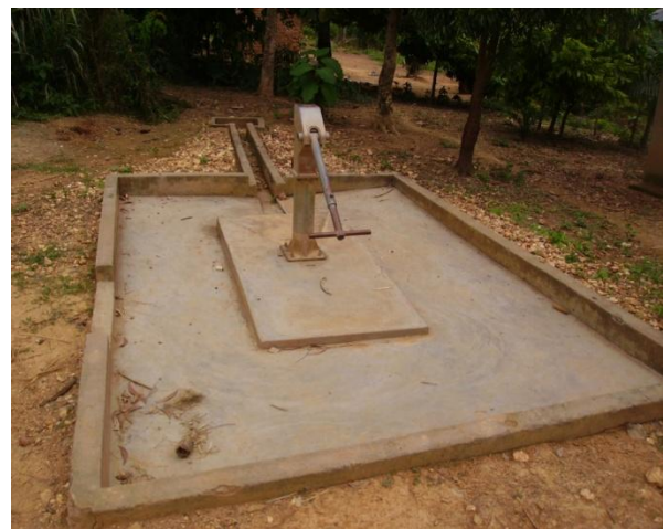
Photo 7. Borehole with hand-pump has no water in the dry season
