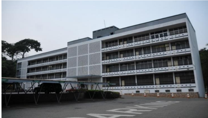
Plate 4.19: Main Administration Block (February 1960)
