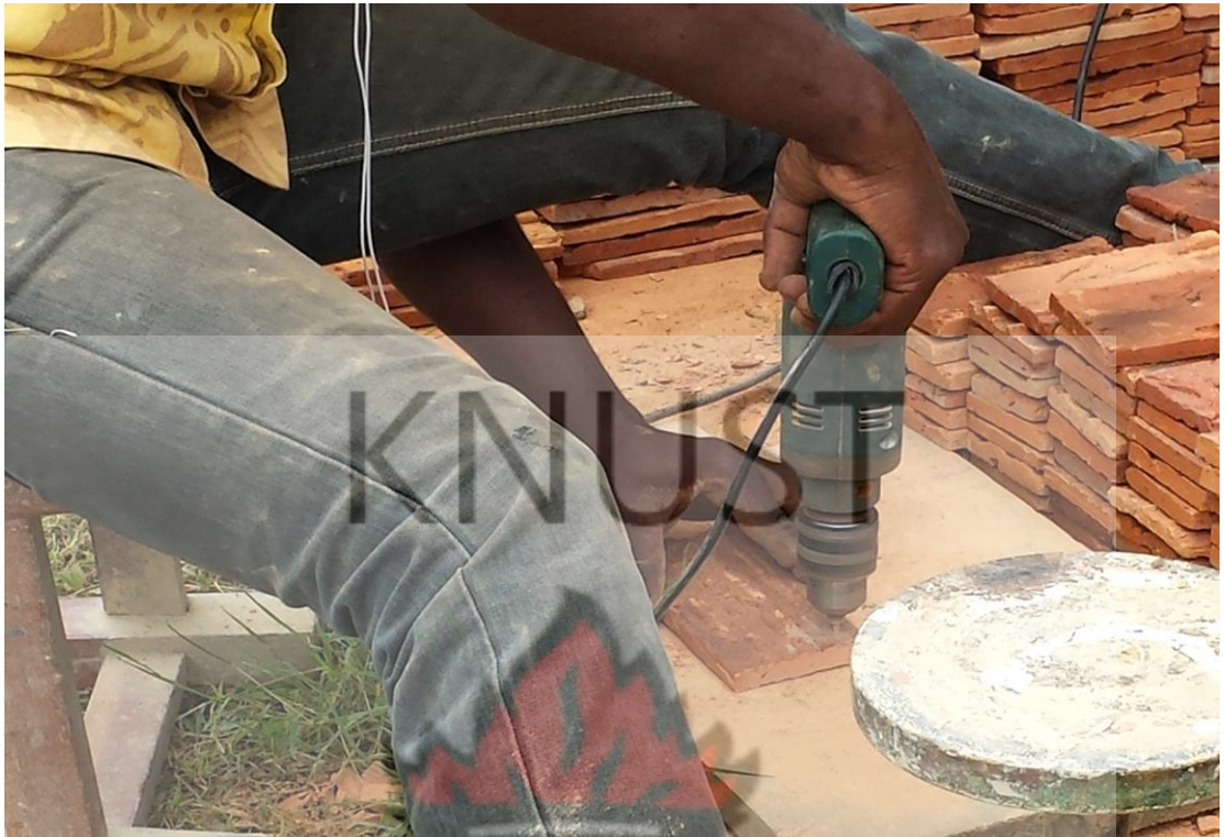
Plate 35: Drilling of holes through tiles
