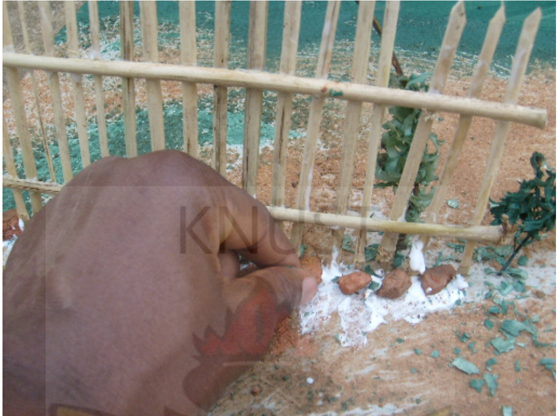
Plate 34: Fixing the fence onto the base.
