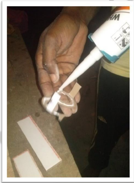
Plate 19: Applying silicone to back of font
