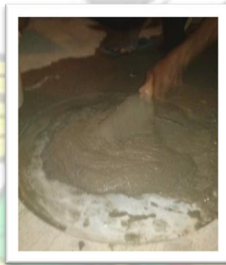
Plate 17: Preparing the mortar
