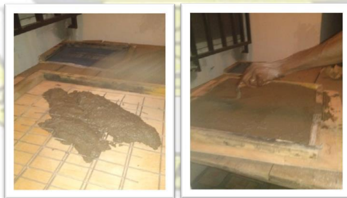
Plate 17: Preparing the mortar
