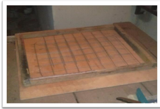
Plate 16: Prepared frame ready to receive the mortar
