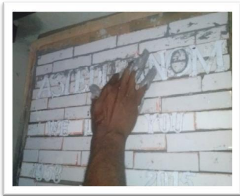
Plate 23: filling the gaps with cement burst
