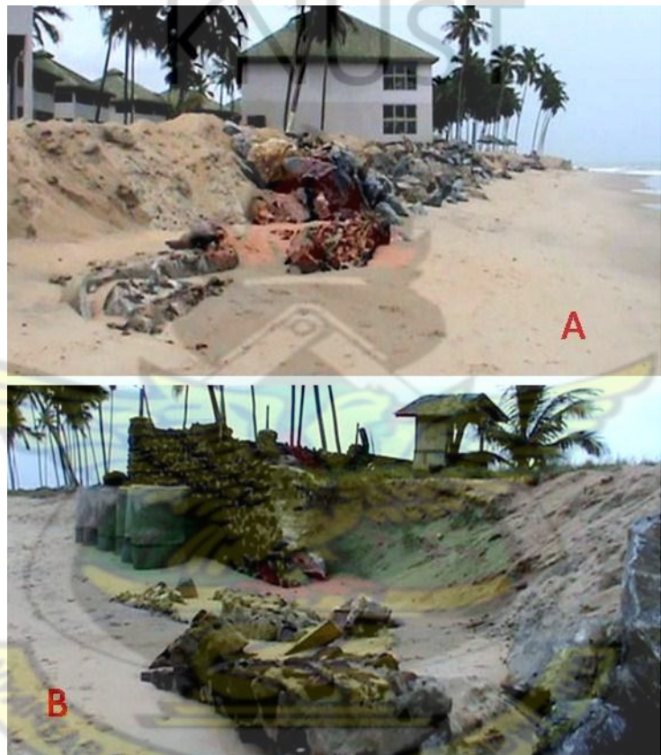
Plate 7 Remnants of various sea defence structures put up to protect the Elmina Bay Resort against sea waves. Source: Fieldwork: June 8, 2012.
