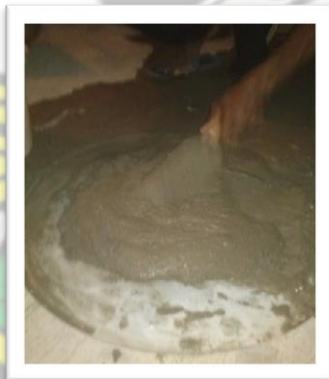
Plate 17: Preparing the mortar
