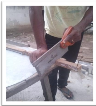
Plate 13: Cutting of wood to the
