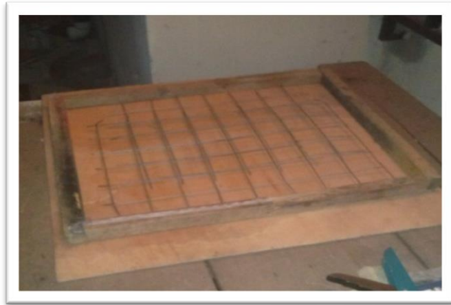
Plate 16: Prepared frame ready to receive the mortar
