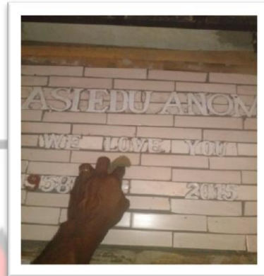
Plate 24: Cleaning debris from the work
