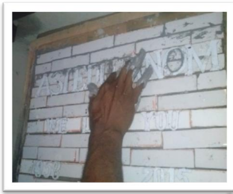
Plate 23: filling the gaps with cement burst
