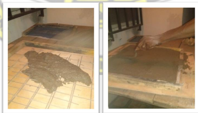
Plate 18: Filling the frame with mortar to receive the tiles
