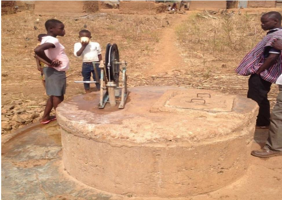
Plate 6.6 A photograph showing a closed hand-dug well with a pulley system.
